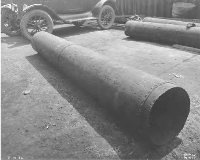
Fig. 2.10 Pits in 16 in. Sheet Iron Water Main in San Francisco's East Bay that failed in 1 month due to leakage of current from electric streetcars. (Photo dated August 10, 1926, Courtesy of East Bay Municipal Utility District.)
