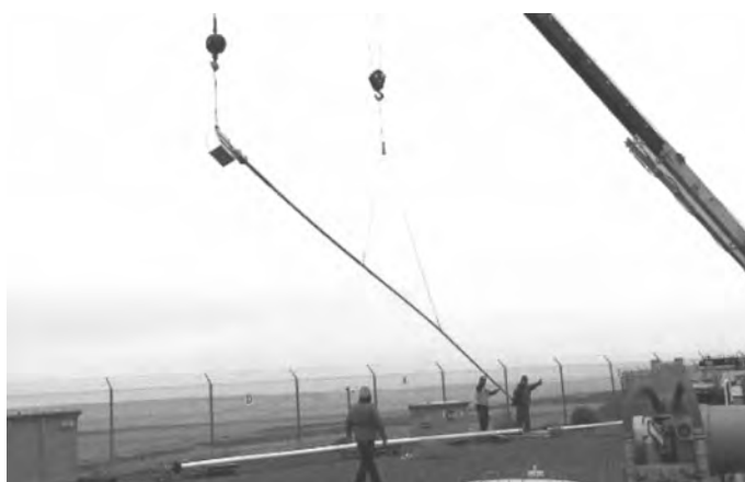
Fig. 4.6 Installation of first full-scale probe into a double-shell tank (DST) at the Hanford site. (Courtesy of HiLine Engineering & Fabrication.)
