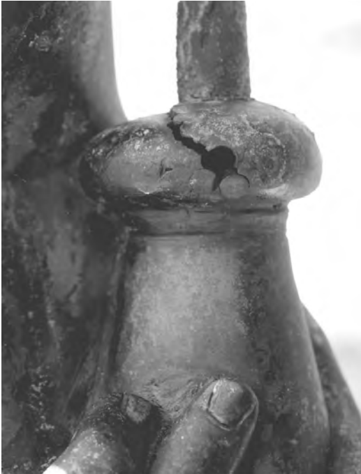
Fig. 2.25 Stress corrosion crack in a bronze monument caused by build-up of rust around a decorative steel rod. (Courtesy Kingston Technical Software.)
